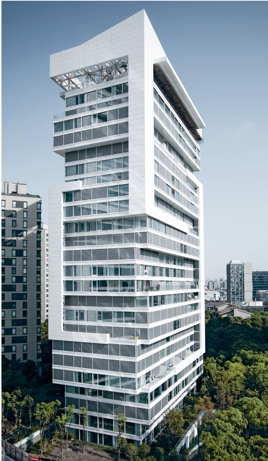
↑ Architect: Dibelius Architekten, Hamburg → Architect: Max Dudler GmbH, Berlin
