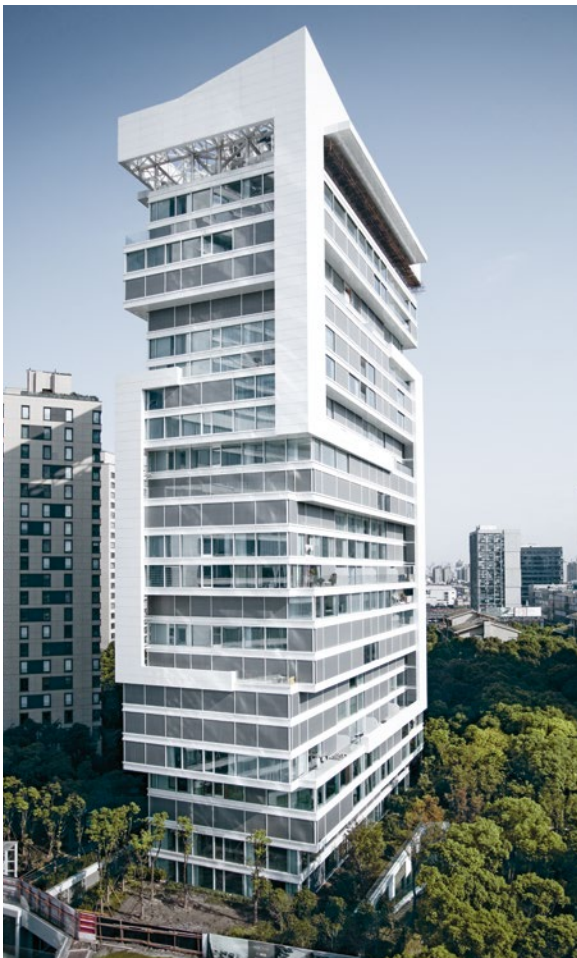
Shanghai, China Two residential blocks with pressure/suction load of 316 kg/m 2 . Maximum noise insulation requirements due to the central location.
